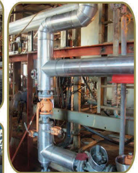
Insulation Work in Smart Village - Gasco
